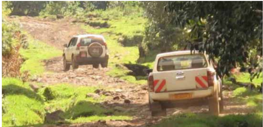
Figure: 2.7 Approach road to Mgahinga Gorilla National Park in poor condition
