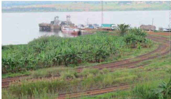
Figure: 2.12 Operational railway tracks by the Nile at Jinja
