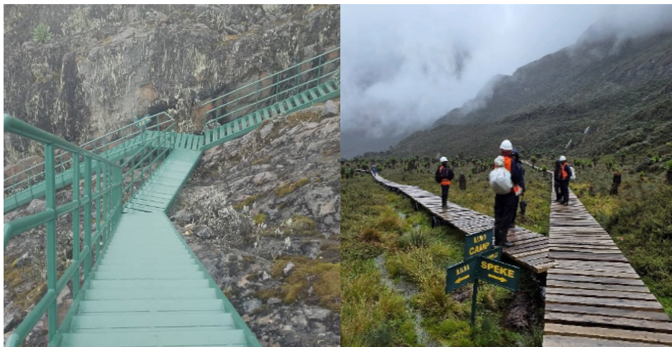
Climbing Ladders and Boardwalks in Rwenzori Mountains, 2026
