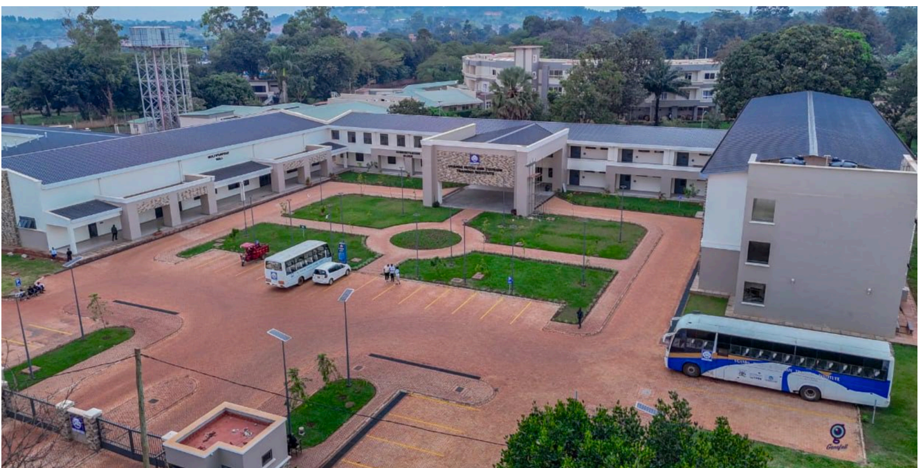
Newly Constructed Admin - Classroom Blocks for HTTC in Jinja, 2026
