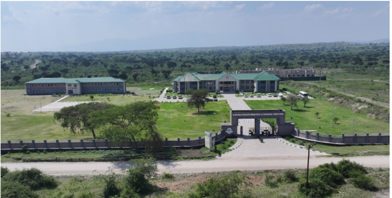
New structures at Uganda Wildlife Research and Training college, 2026
