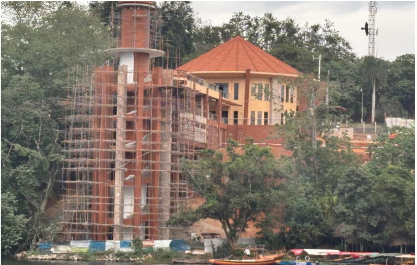
Source of the Nile Pier under Construction, 70% level of completion.
