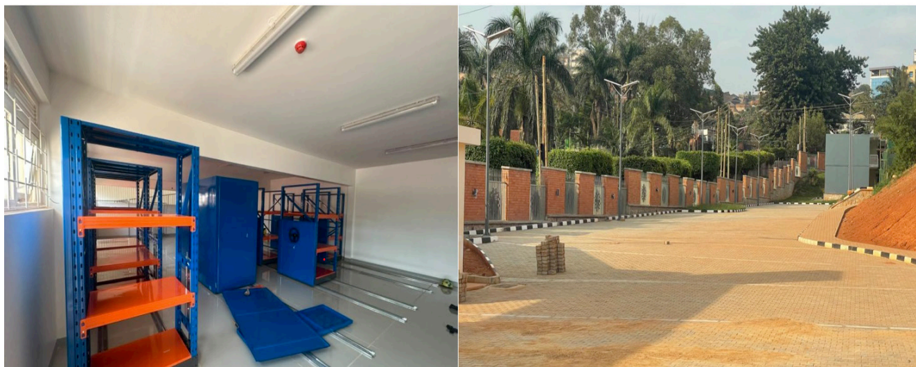
Source of the Nile Pier under Construction, 70% level of completion.
