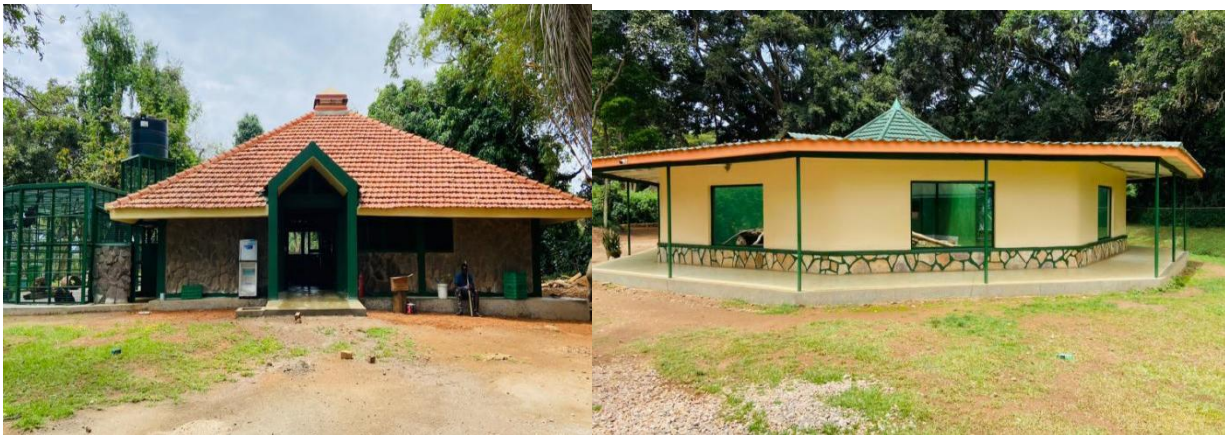
Renovated chimp house
