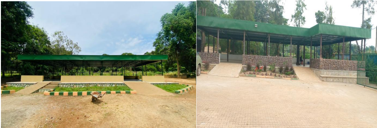
Completed visitor shades
