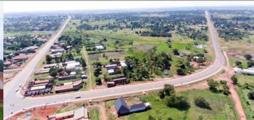
Civil works for upgrading of LOT 1- Tirinyi-Pallisa-Kumi Road (67 km)
