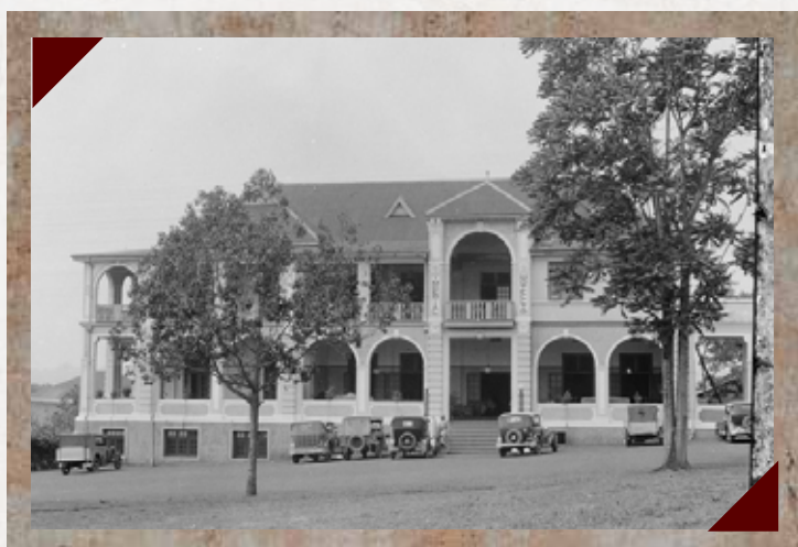
Lumumba Hall officially opened in 1970's
