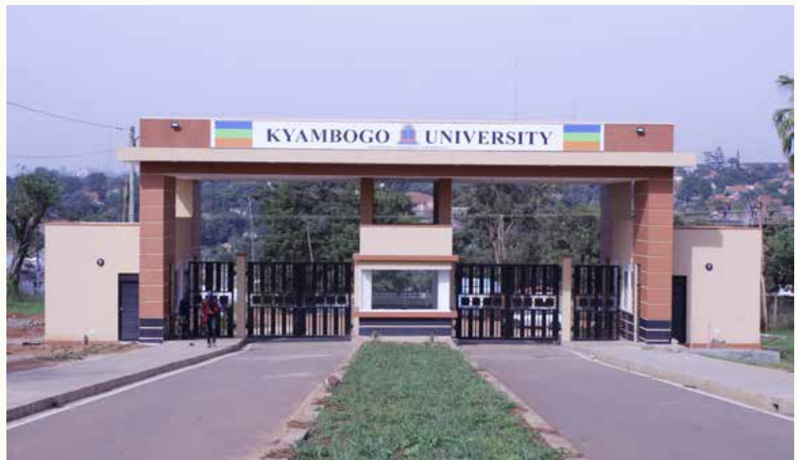
Kyambogo University main gate
