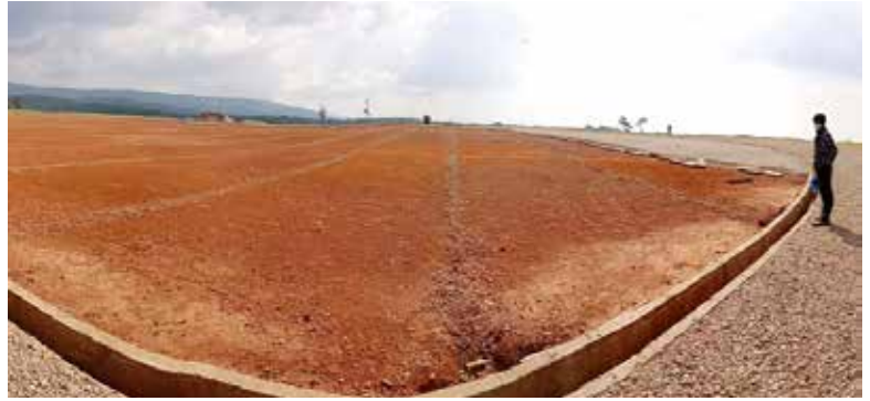
National High-Altitude Training Centre at Teryet: The Artificial Football/ Rugby Turf Field is at 80 per cent completion.
