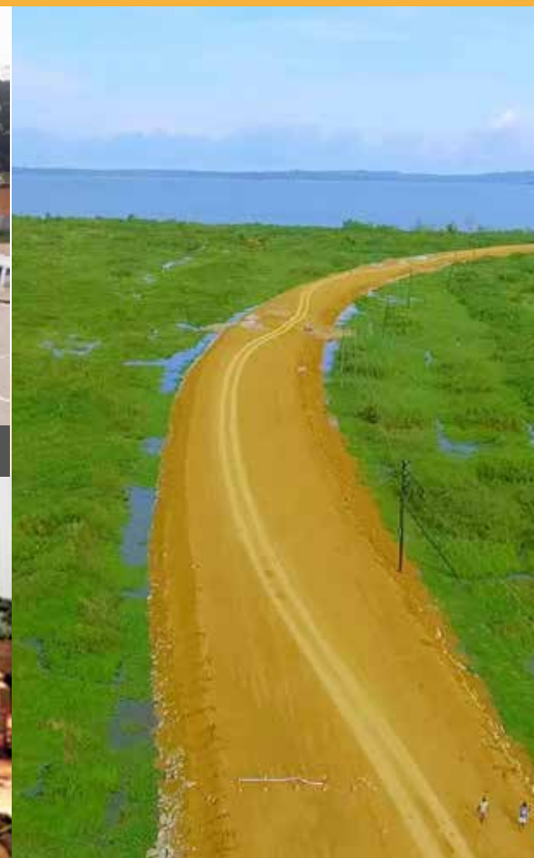
Civil works for upgrading of Masaka-Bukakata road (41 km)
