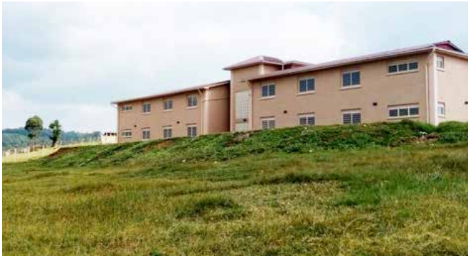
Construction of the Hostel Block at the National High-Altitude Training Centre in Teryet is at 98 per cent completion.
