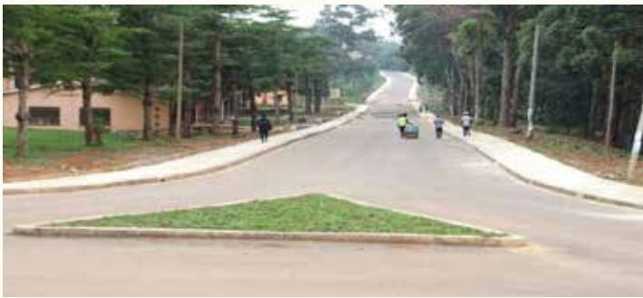
Some of the newly constructed roads at Kyambogo University
